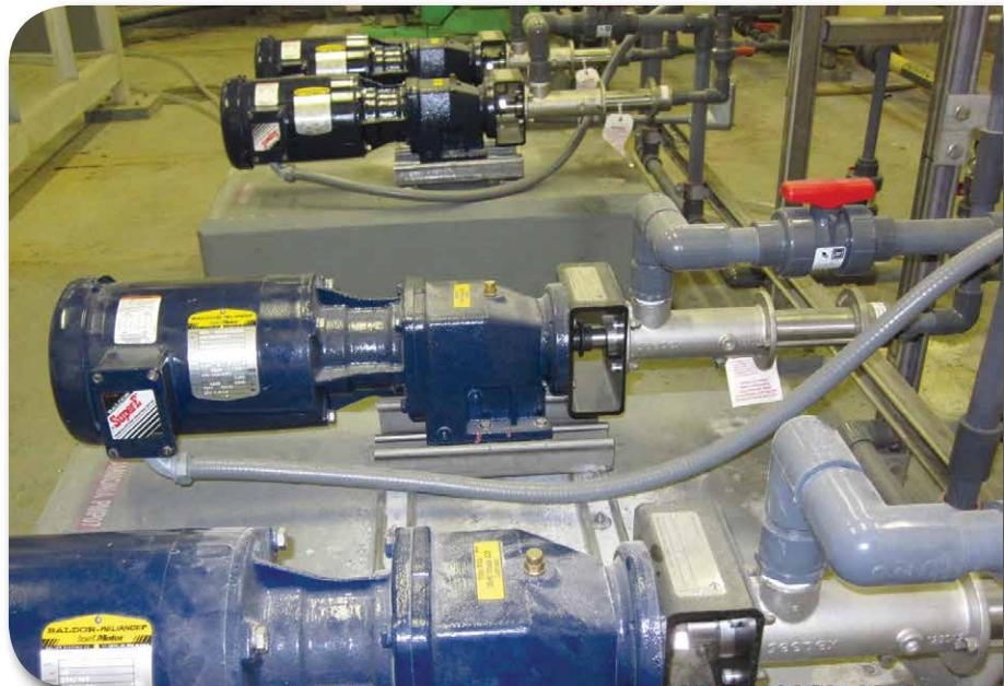
workload, Branch looked for a model with a long lifecycle to extend savings over time. Stuart Taylor, a sales engineer for Tencarva Machinery in Chesapeake, Virginia, recommended the progressive cavity metering pumps. "The seepex titanium fitted MD pumps are a tight little package," he explains.
